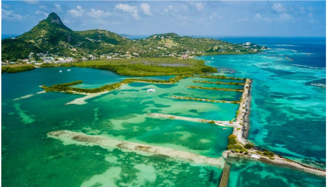
Aerial view of Ashton Lagoon during excavation of gap #2, November 2017. Photo credit: Arthur Daniel.
