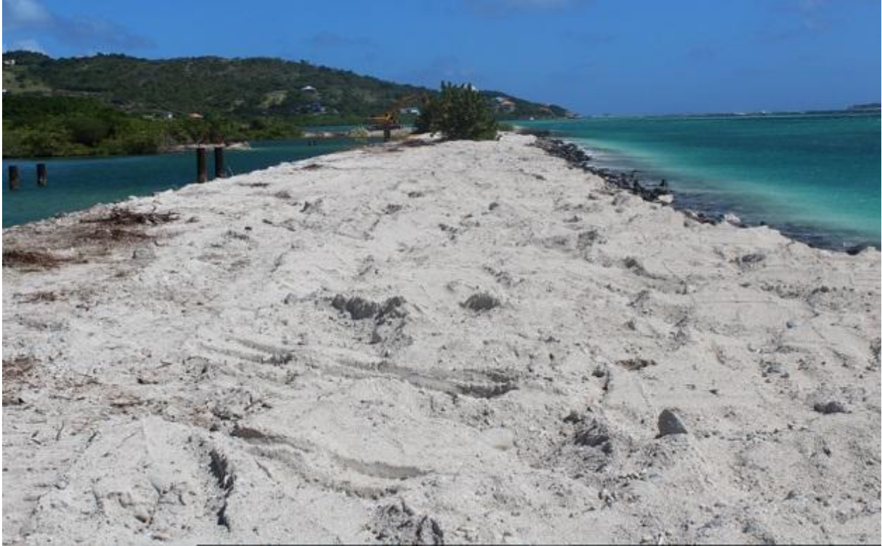
Above and below: The main causeway at the end of Phase I. The excavated sand has been placed and graded on the seaward side.
